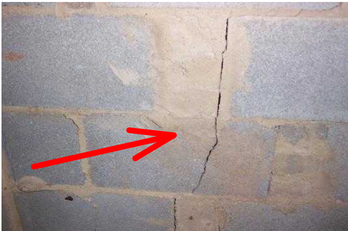
Foundation crack
